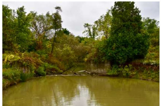
McKenzie Creek just downstream of the dam on Indian Line.
